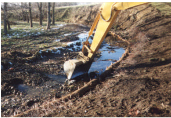
Project site during construction.
